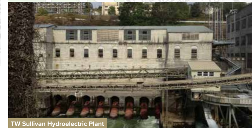
TW Sullivan Hydroelectric Plant
